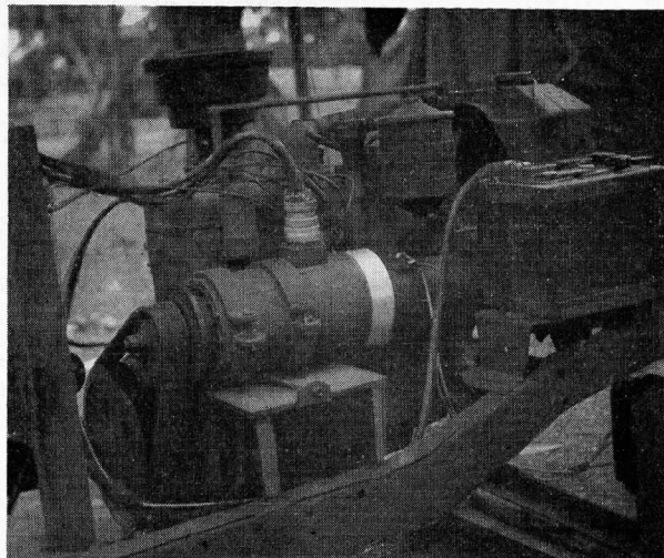
IMPROVED 24-VOLT GENERATOR CONSTRUCTED IN SWPA BY SIGNAL CORPS MEN OF AN AIR SERVICE COMMAND.
