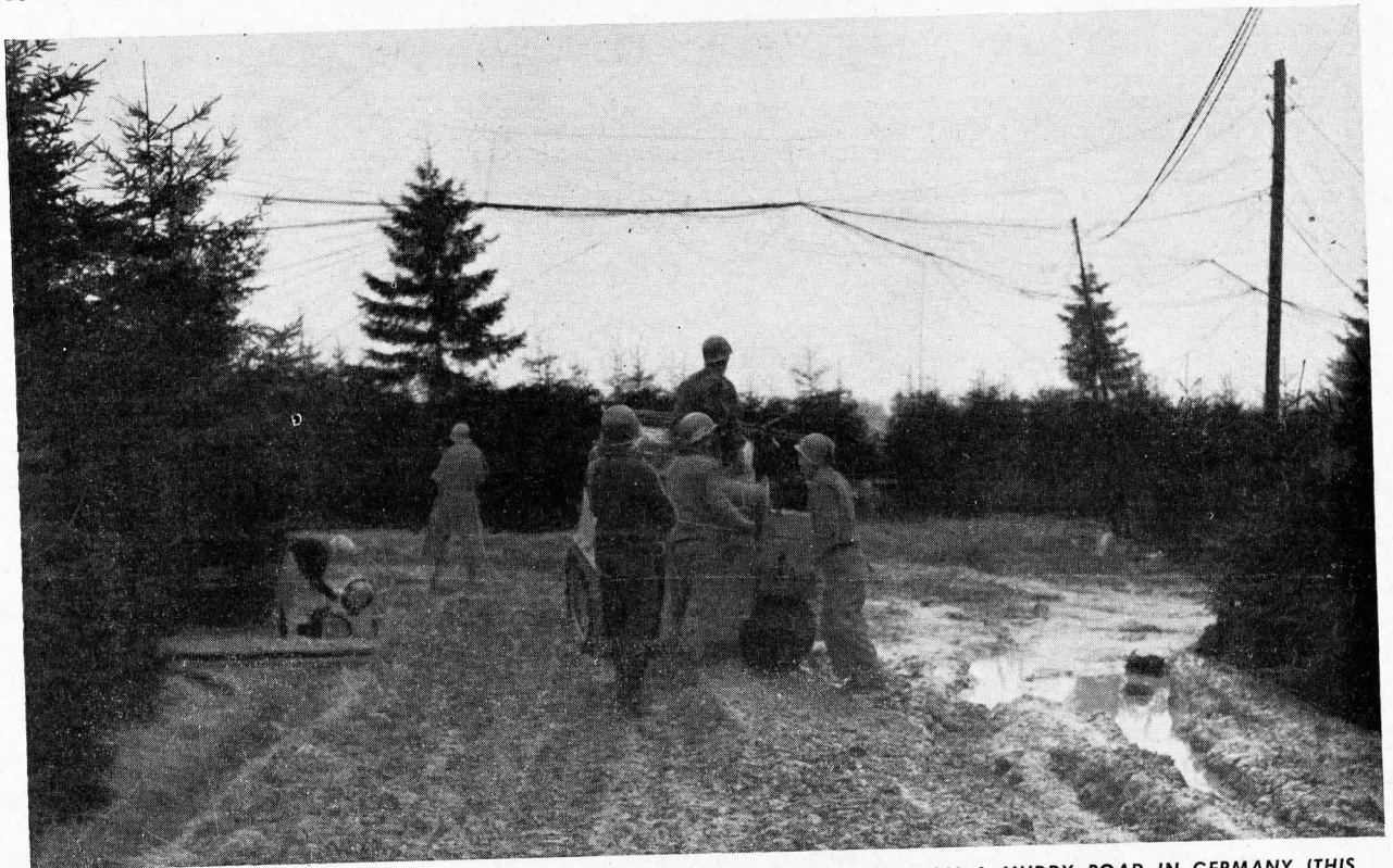
A WIRE TEAM OF THE 56TH SIGNAL BATTALION USING A "WEASEL" TO LAY WIRE ON A MUDDY ROAD IN GERMANY (THIS PICTURE WAS TAKEN IN MID-FEBRUARY).
