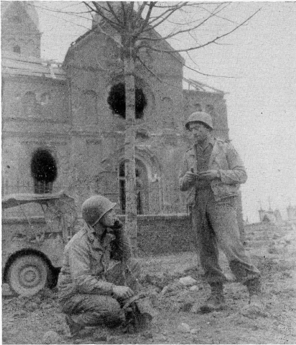
SIGNALMEN OF THE 1ST SIGNAL COMPANY REPAIRING A LINE IN GERMANY LATE IN FEBRUARY
