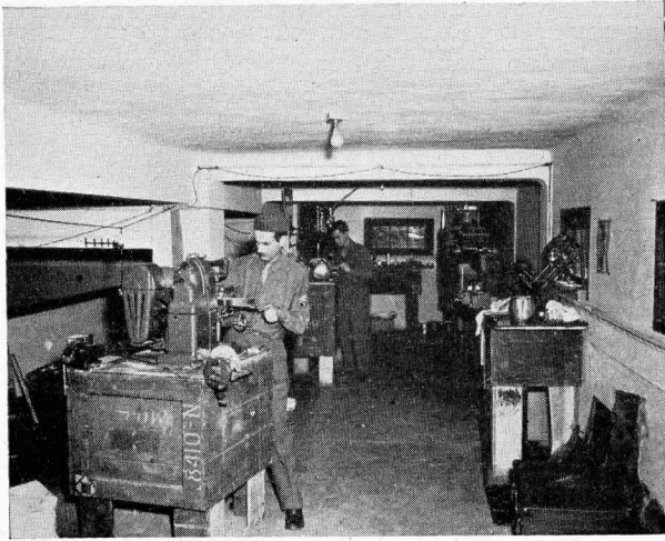
"THE MAINTENANCE SECTION WAS SET UP ON A BALCONY."
