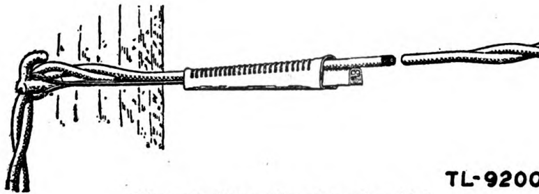
Figure 3. Drop wire clamp installed.
