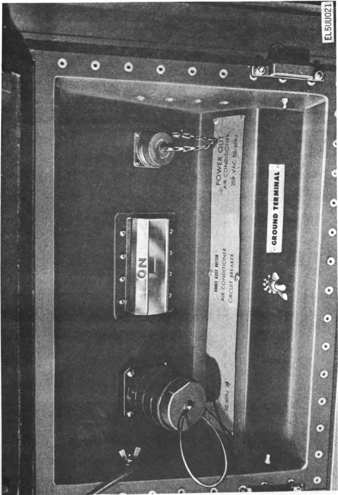
Figure 1-15. AC Power Entrance Panel.
