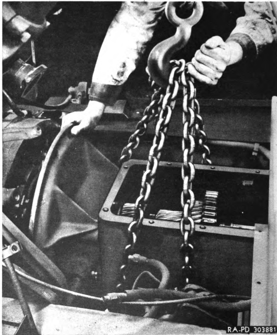
Figure 96—Removing Transmission
