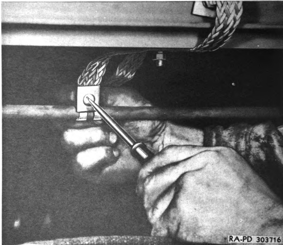
Figure 206—Disconnecting Hood Bond Strap
