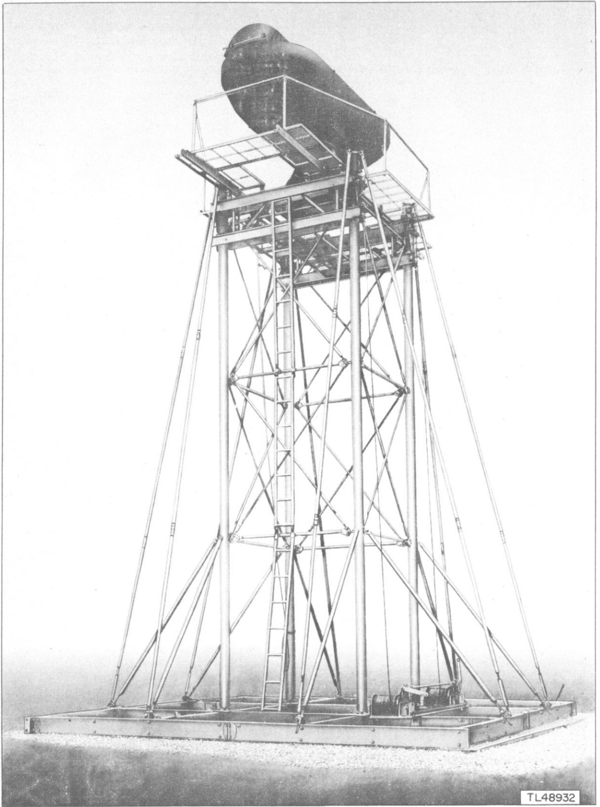
Figure 2-34. Tower completely erected.
