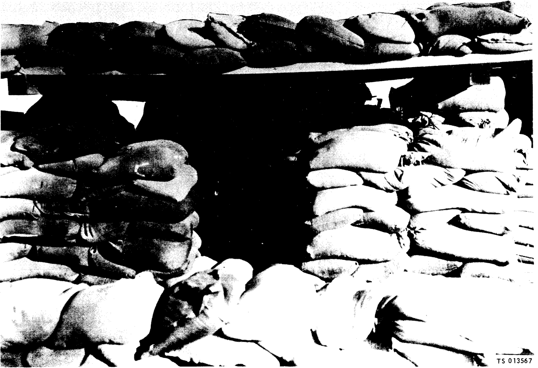
Figure 4-5. Revetment, front view.
