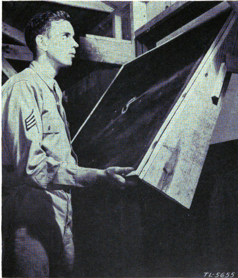
FIGURE 44.—Attaching tar paper shades.
