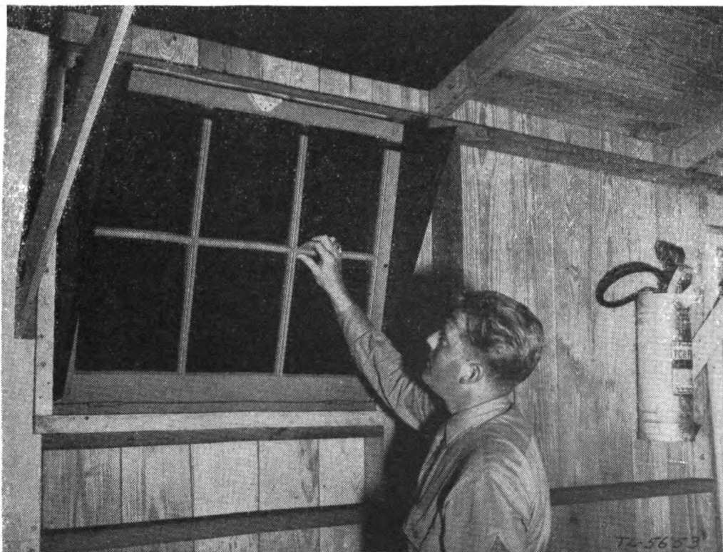
FIGURE 42.—Painted windows with ventilation blinders.
