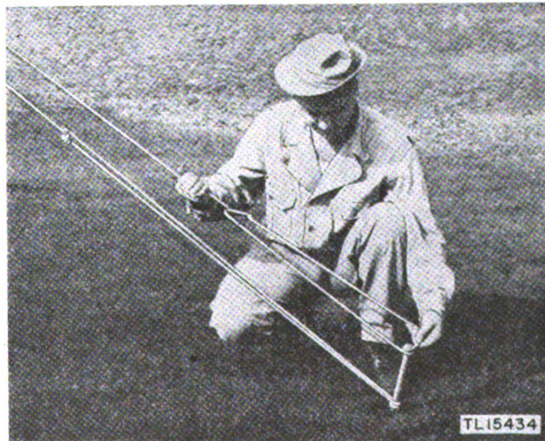
Figure 14. Looping hoist rope over stake.
