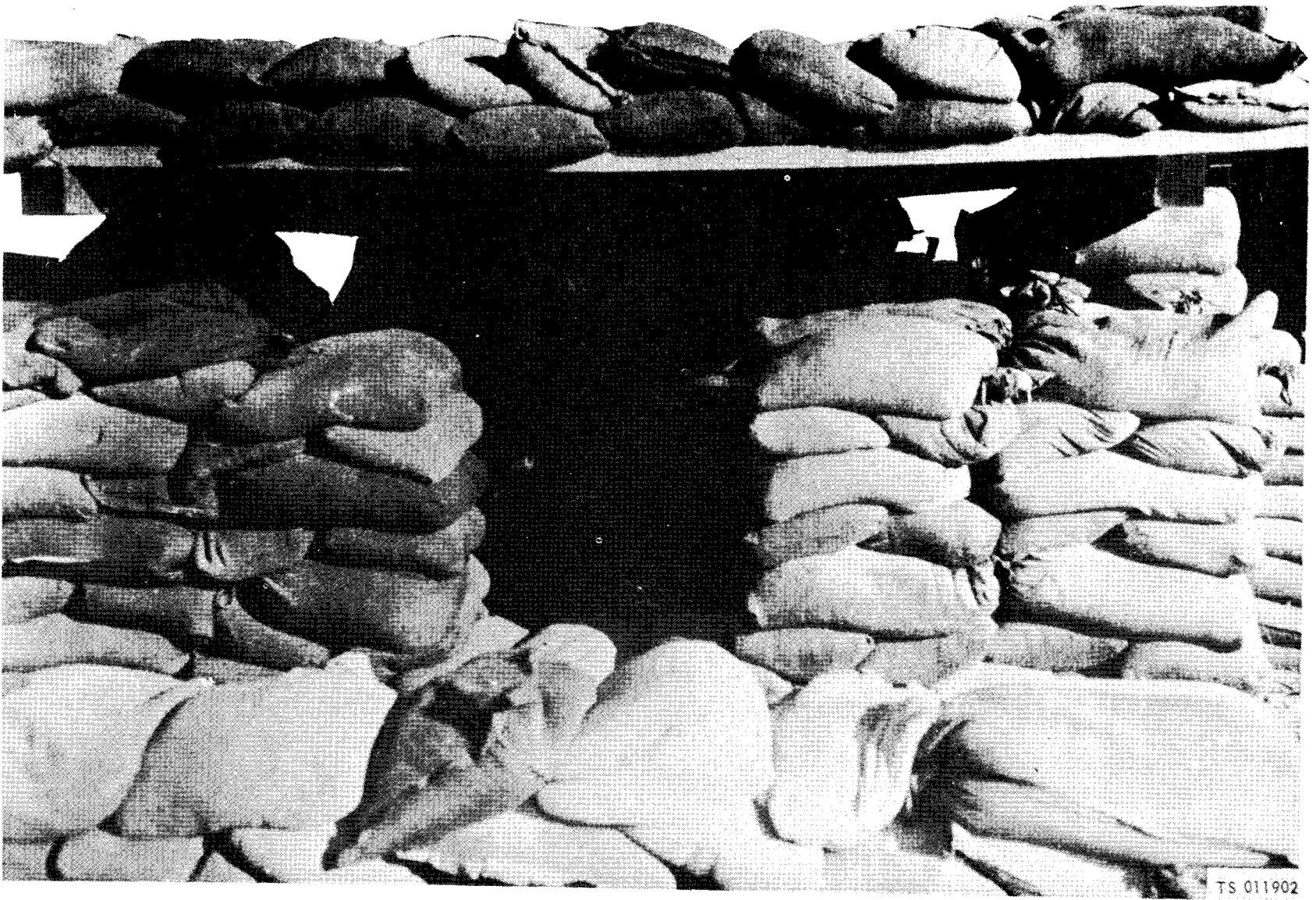
Figure 4-8. Revetment, front view.
