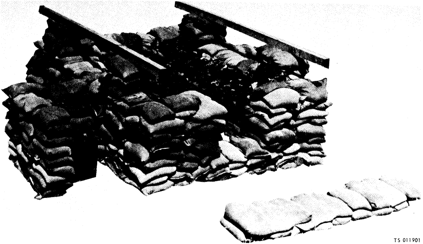
Figure 4-7. Revetment, perspective without roof.
