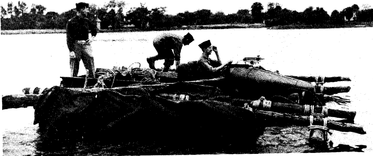
ACTUAL FERRYING OF VEHICLE ACROSS STREAM
