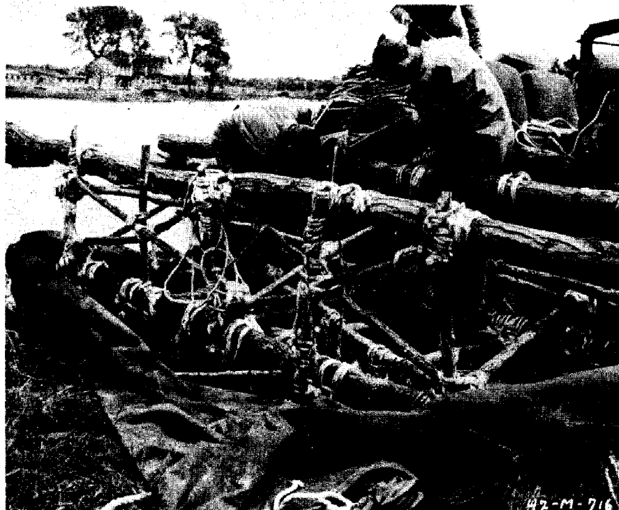
FRAMEWORK BEING CONSTRUCTED FOR A \frac{1}{2} -TON 4 X 4 TRUCK
