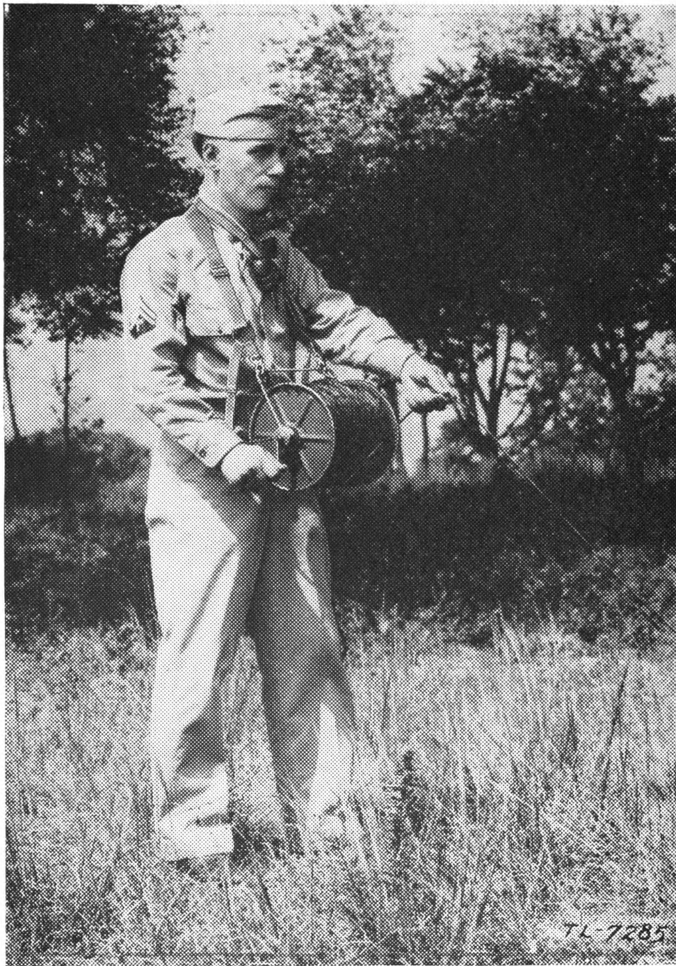
Figure 4. Recovering wire with Reel Equipment CE-11.
