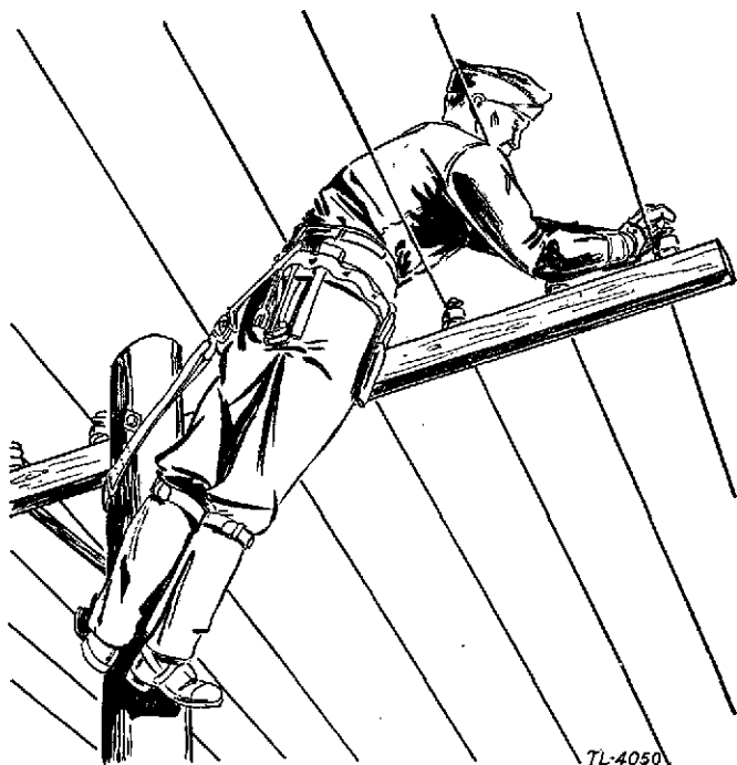
FIGURE 75.—Working on outer wire of cross arm.
