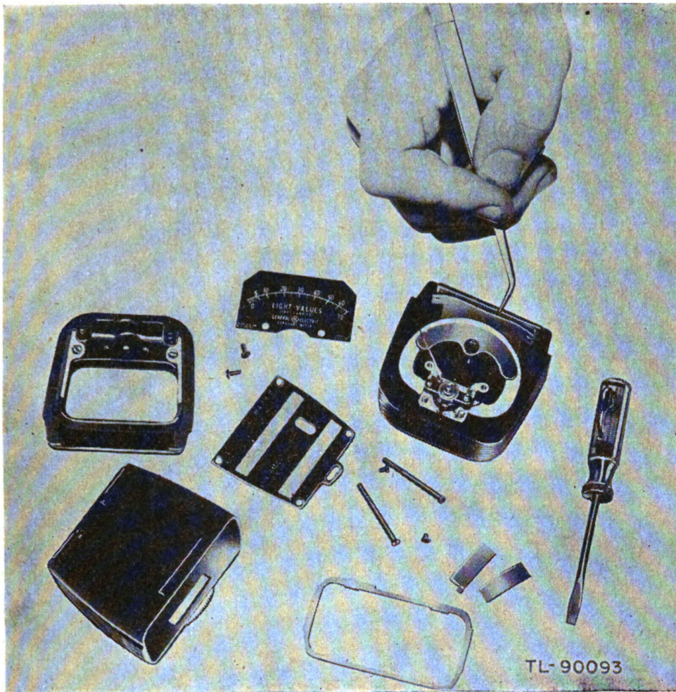
Figure 22.—Photoelectric cell of Exposure Meter PH-77-C General Electric DW48.
