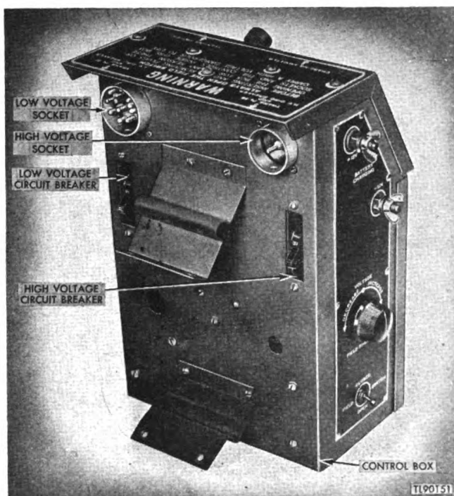
Figure 68. Control box for Power Units PE-49-F and PE-49-G—rear view.
