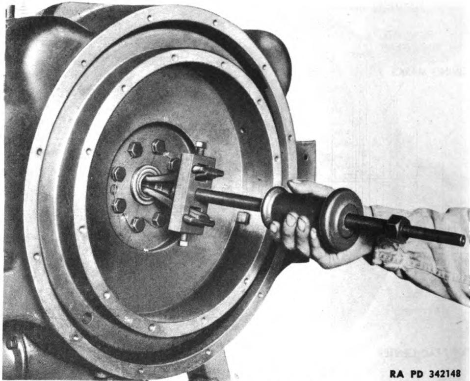
**Figure 53—Removing Clutch Pilot Bearing, Using Puller (41-P-2957)**
