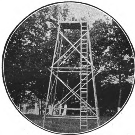
A PORTABLE TOWER CARRIED BY FIELD TROOPS IN SECTIONS AND ERECTED IN A FEW MINUTES, PROVIDING AN ELEVATION FOR OBSERVATION AND VISUAL SIGNALING
