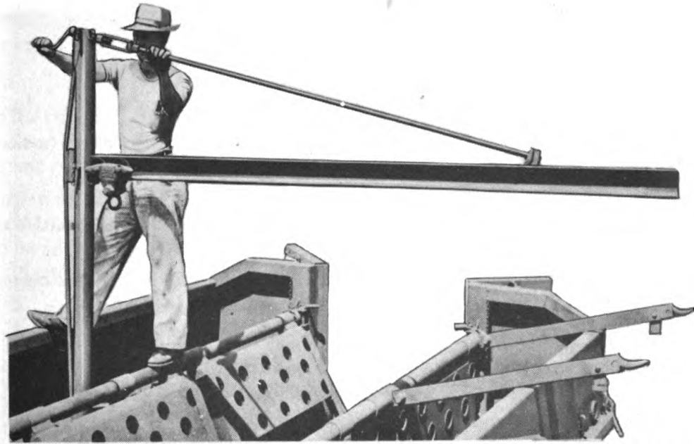
Figure 44 — Adjusting Boom To Proper Level
