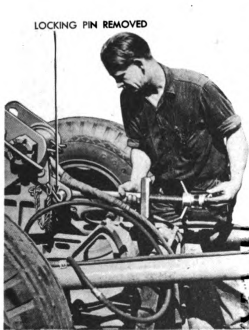
A—REMOVING EYE BOLT
