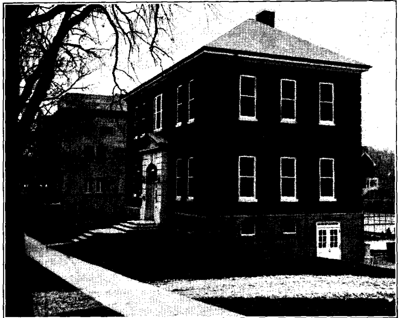
Communication Building, Fort Leavenworth.
