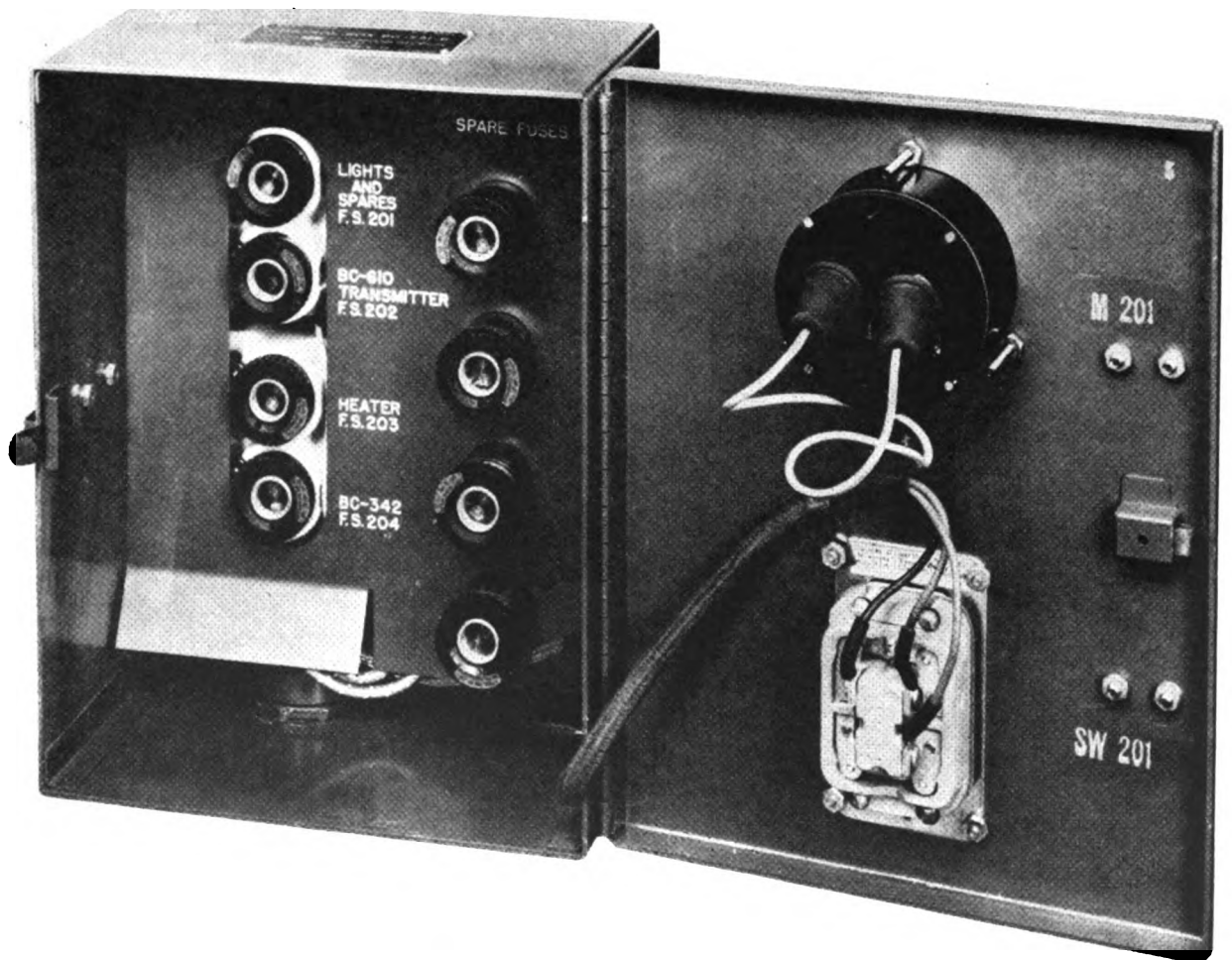
FIGURE 17. CONTROL BOX BC-731-(*), INTERIOR.
