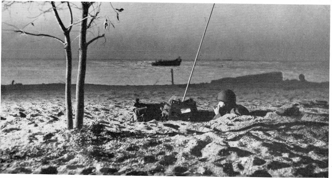
BEACH RADIOMEN DIG IN QUICKLY AND MAINTAIN CONTACT WITH LANDING CRAFT THROUGH THE SCR-610.
