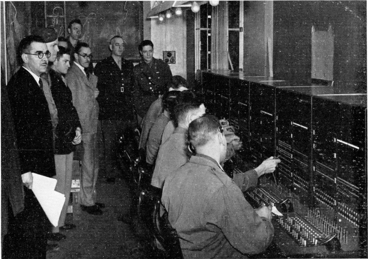
BRITISH GPO ENGINEERS AND U. S. ARMY OFFICIALS AT THE OPENING OF A NEW SWITCHBOARD "SCMEWHERE IN ENGLAND."
