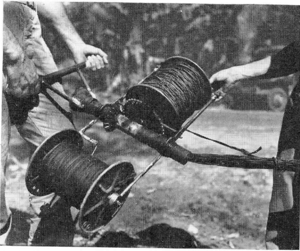
CABLE BINDER DESIGNED BY SIGNALMEN OF THE 37TH DIVISION.
