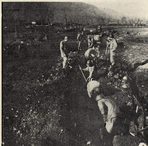
OPENING A CABLE TRENCH IN ITALY FOR REHABILITATION.
