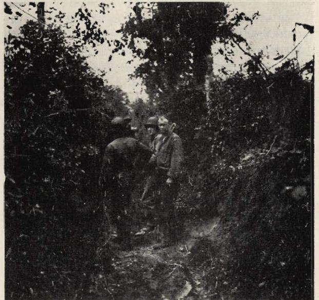
STRINGING WIRE ALONG THE HEDGEROWS OF NORMANDY.
