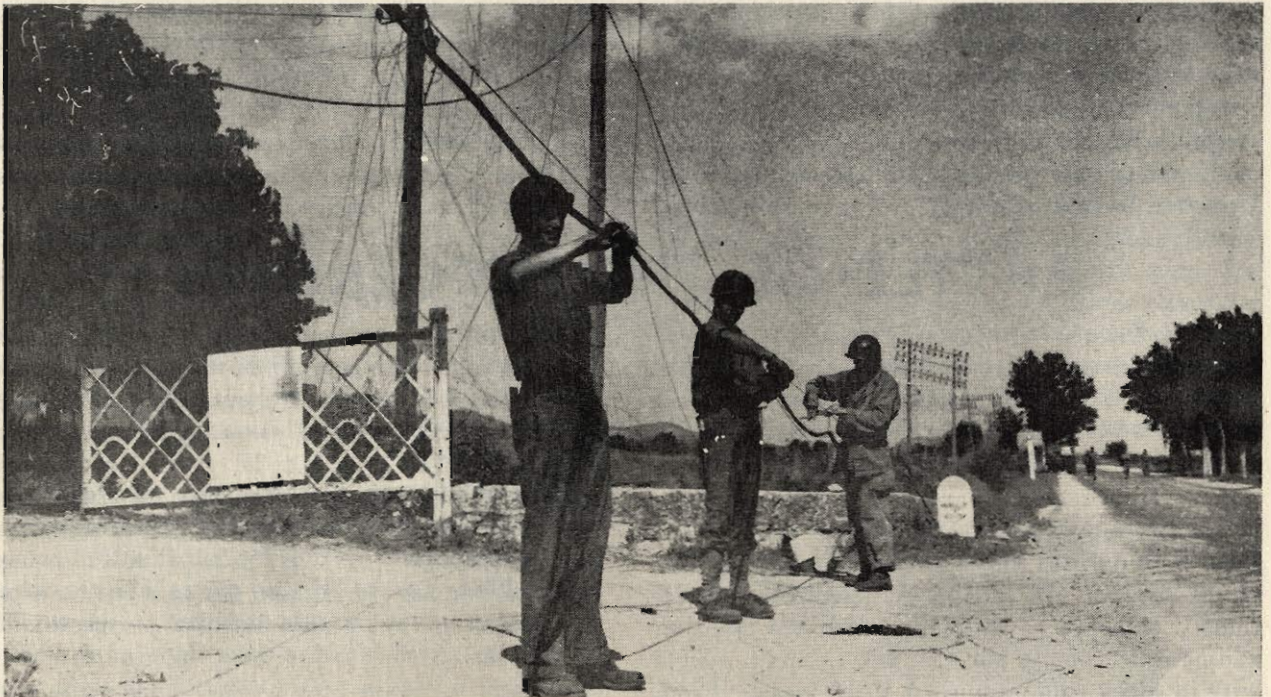
SEVENTH ARMY SIGNAL MEN SETTING UP SPIRAL-FOUR CABLE ON MESSENGER IN THE BRIGNOLES AREA OF SOUTHERN FRANCE.
