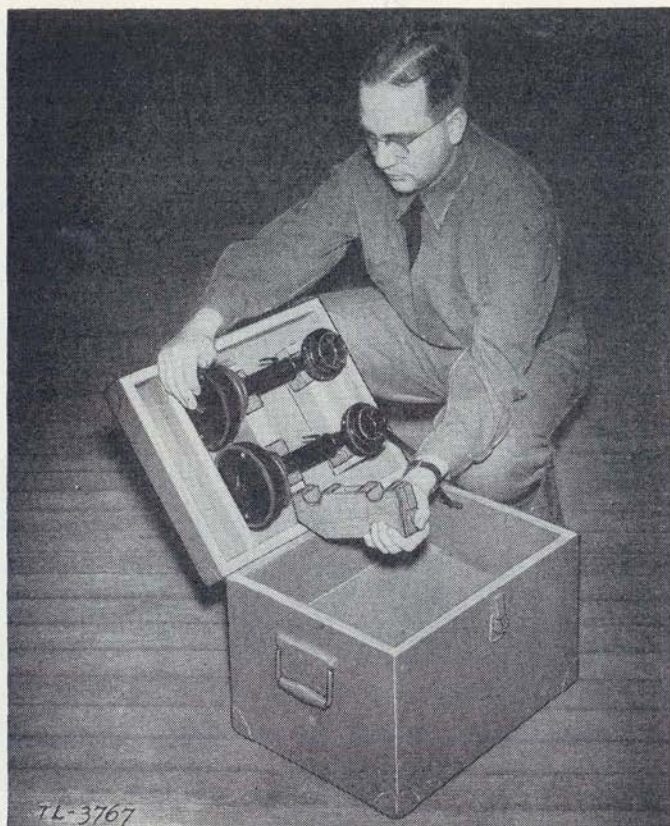
FIGURE 6.—Chest CH-55-A opened to show how microphones T-32 rest in cover.
