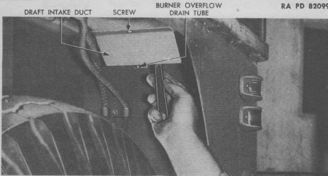
Figure 135—Removing Draft Intake Duct
