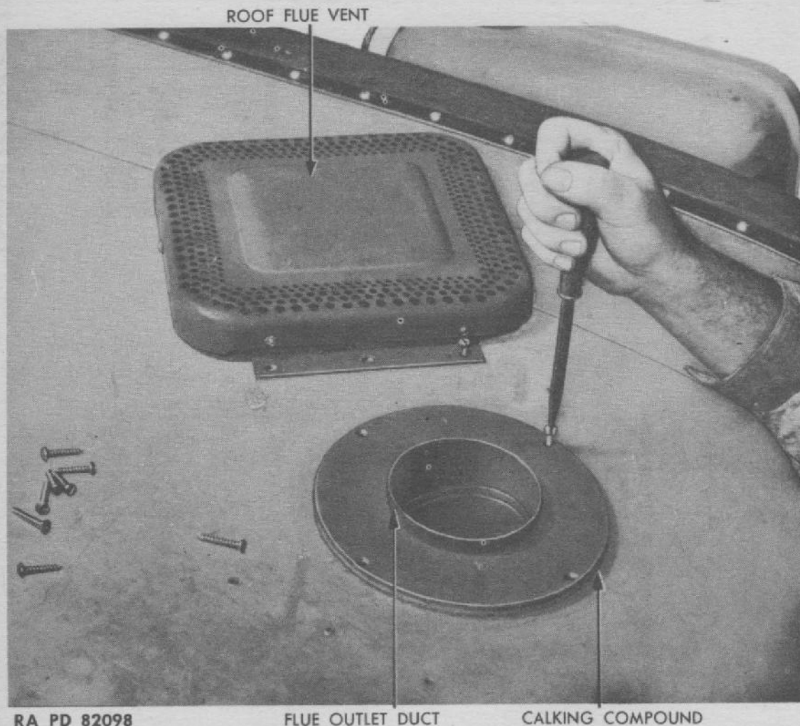
Figure 133—Removing Vent and Flue Outlet Duct
