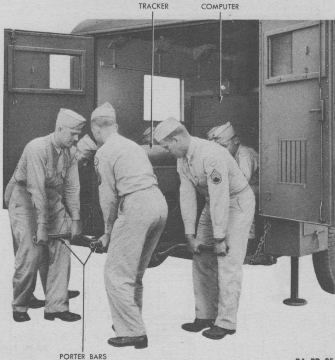
Figure 104—Installing Tracker
