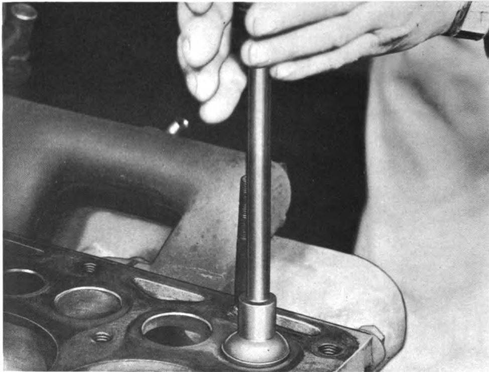
Figure 118—Grinding Valves
