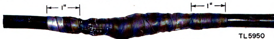
Figure 38. Rubber tape applied to splice.
