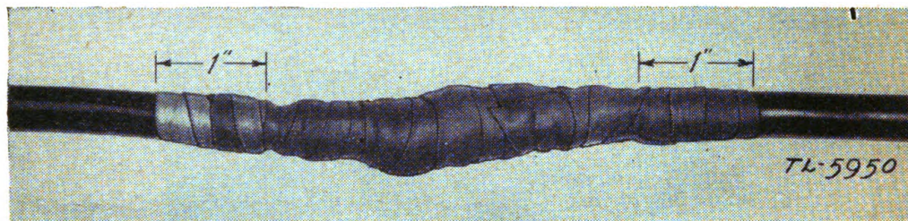
FIGURE 20.—Rubber tape applied to splice.
